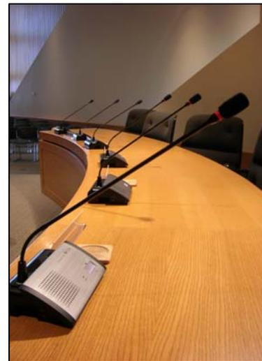
TOA's TS-900 Series has the capability of being monitored by Creston control panels, which the Town of Whitby has been using. Creston's control panel allows the chairperson to be able to fully control all conferencing functions, including microphone functions such as mute on/off. The Town of Whitby can also expand the system to include voting (which is currently not being used). The conference system integrates nicely with the other products selected to work within the council chambers.
