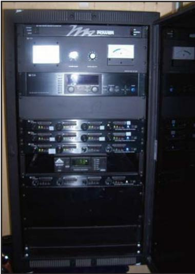
– Ambient Noise Control Modules. There are three microphones to monitor the noise levels in three areas of the mall. These areas include; the food court; central court; and end court (an area for special events, kiosks, Santa, etc.) where high traffic and excessive noise exist. The Ambient Noise Control Module allows the PA system to be monitored for noise levels and allows for appropriate adjustments to be made to the PA system.
